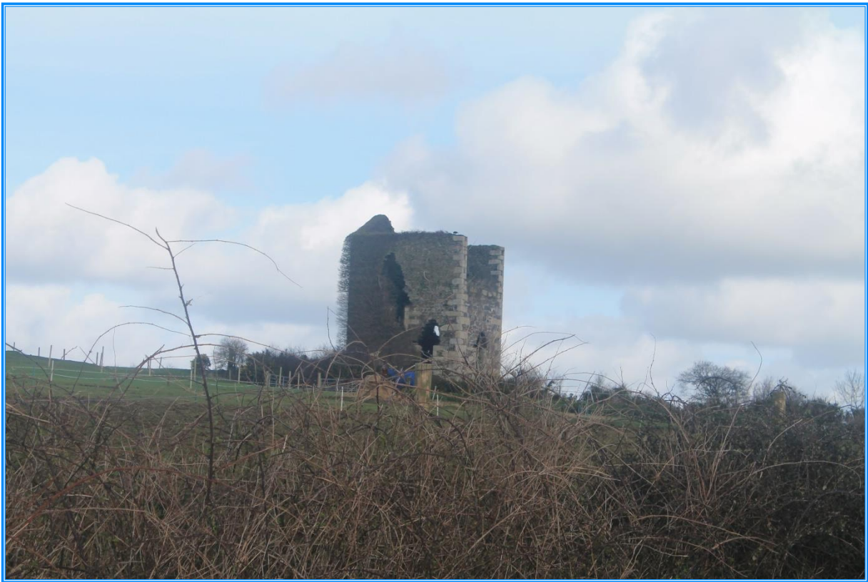
Austin's Shaft Engine House
