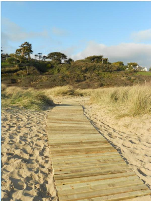
Example of a removable access structure (Source: <http://lizardandpenrose.blogspot.co.uk/2012/03/under-boardwalk.html>; link correct when accessed on 29<sup>th</sup> July 2016).
