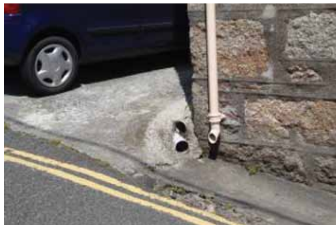
Private roof and surface water directed onto the highway
