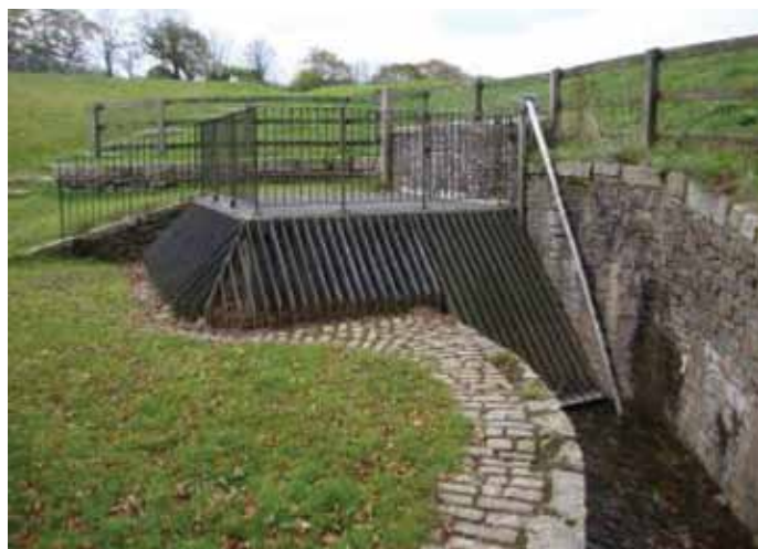
Outlet structure in an area designed to flood
