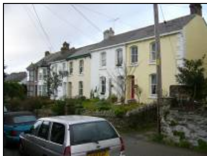
Villa-type terrace development, North Street
