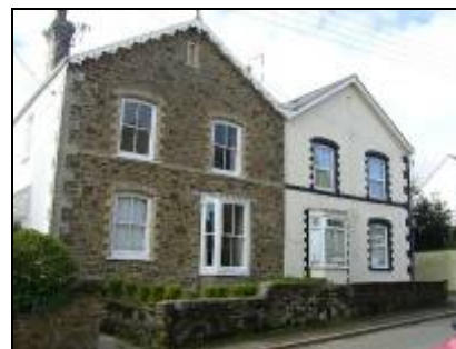
Incremental loss of architectural detail affects character
