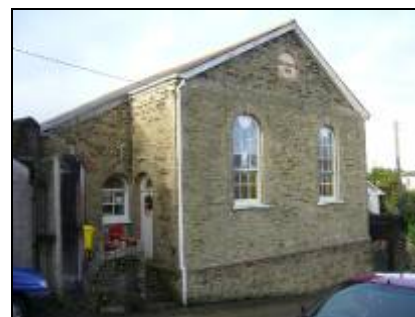
Former Wesleyan Sunday School, Well Street
