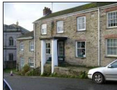
Substantial columns survive from the former Commercial Hotel
