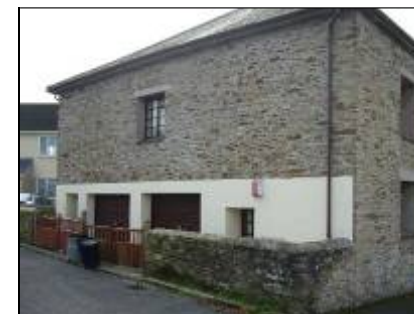
Unsympathetic conversion of former Bible Christian Chapel
