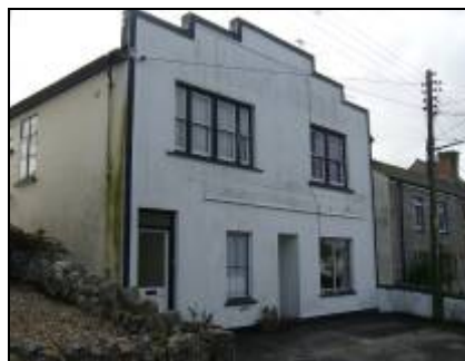
20 th century art deco inspired building, North Street
