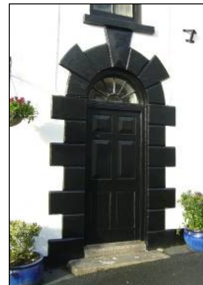
Notable doorways include this impressive example in Fore Street with applied stucco quoins and vousoirs, fanlight and panelled door
