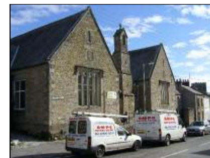
Former National School, 1840s
