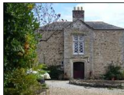
Former Vicarage, early 19 th century Tudor- Gothic architecture
