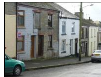
Cottage rows tightly flank the pavement edge in Fore Street
