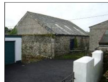
Surviving barns or industrial buildings to the rear of Fore Street
