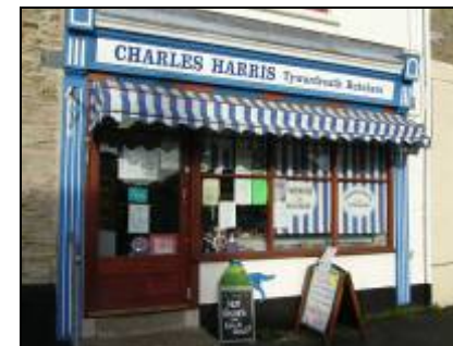
Elements of a historic shopfront survive, Church Street
