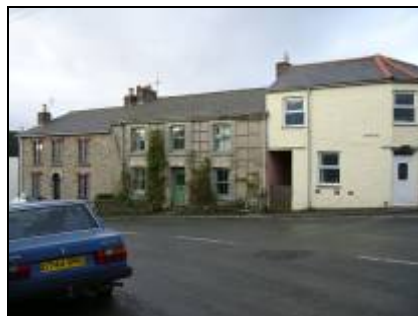
Double fronted houses, Fore Street
